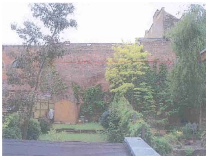
Views from Holmesdale Road
